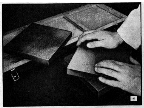
Fig. 2 Refinishing Lapping Blocks
